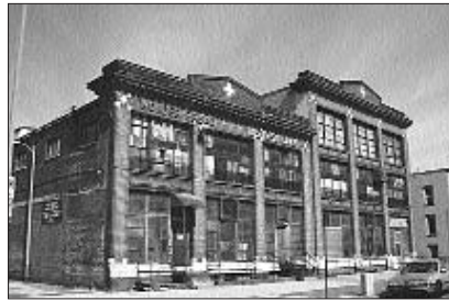
photo—Michael K. Wilkinson—The InTowner
