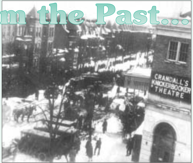
Scores of onlookers gathered along 18th Street on the morning following the collapse of the theater's roof.
