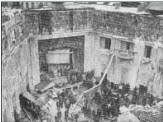
Within the theater, now open to the sky, the devastation was total.
