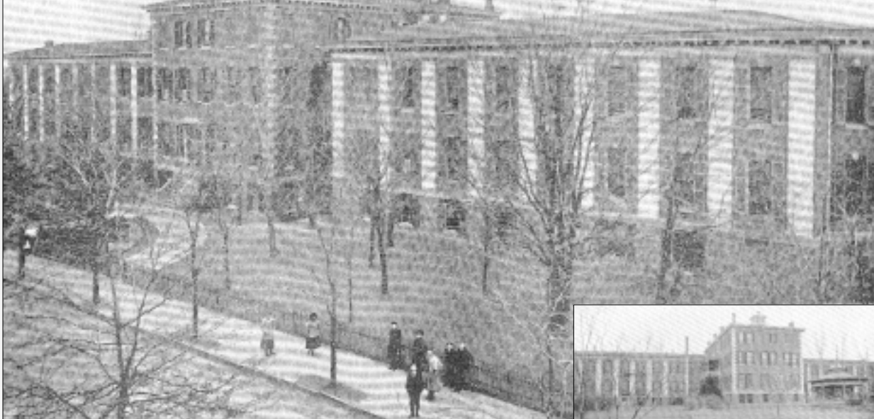
The Children's Hospital of Washington was incorporated in 1870, and maintained a small wood frame building at 13th and F Street until it built, in stages, this large institution facing 13th Street between V and W Street, beginning in 1878. Today the site is home to the Harrison Square townhome development.
